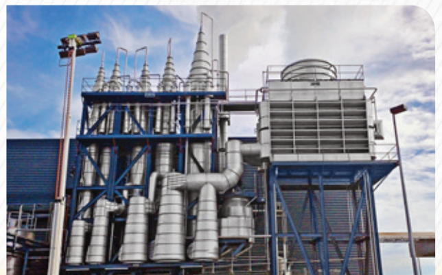
TASTE ® /WASTE installed at Garcia Carrión, in Spain
