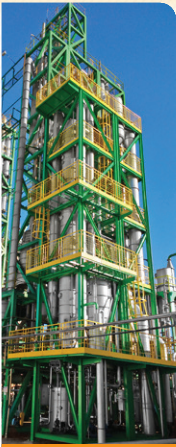
Evaporator ENET with D'Oiler installed in Tropfruit in Estância/SE - Brazil
