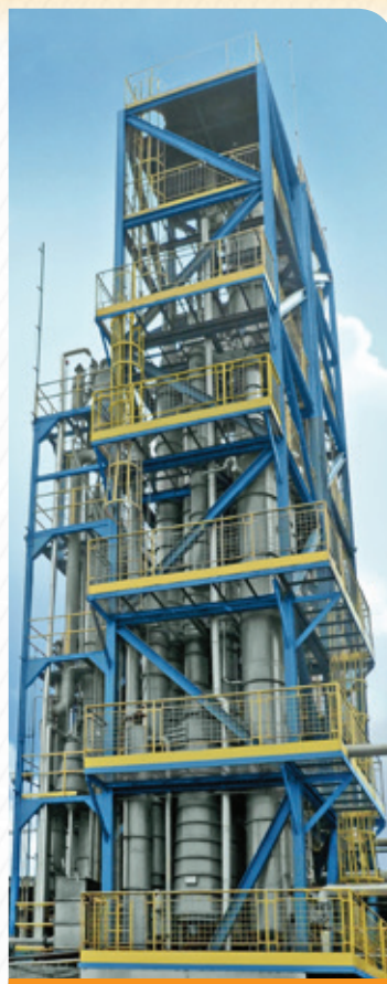
Evaporator ENET with D'Oiler installed in Maratá Sucos in Estância/SE - Brazil
